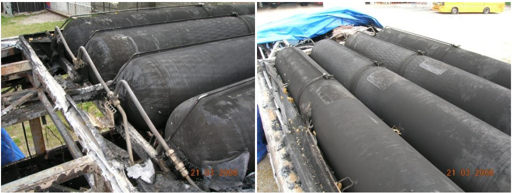
Figure 6. These CNG cylinders were prevented from failing by PRDs which were successfully activated in a fire
