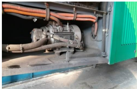
Figure 4. Compressor, steering pump
