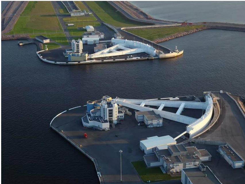
Figure 1 Navigation structures C-1
