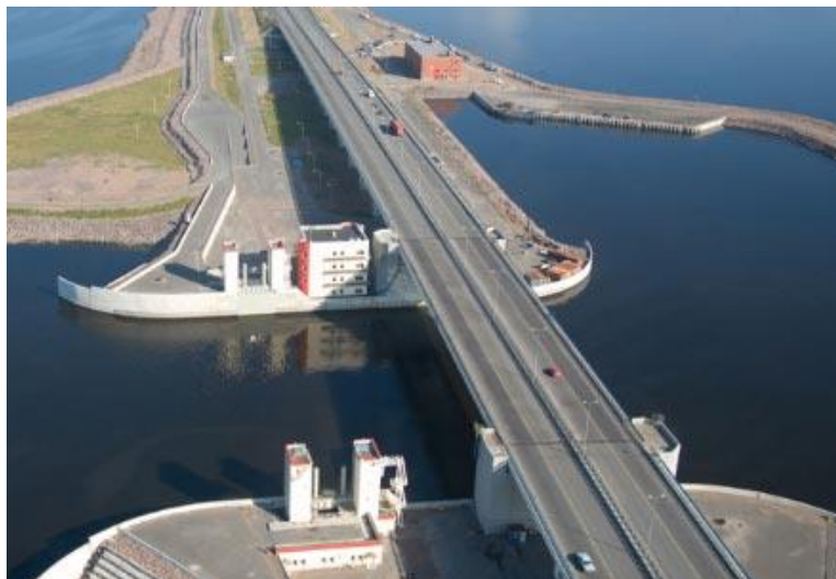
Figure 4 Drawbridge with ship-passing structure C-2
