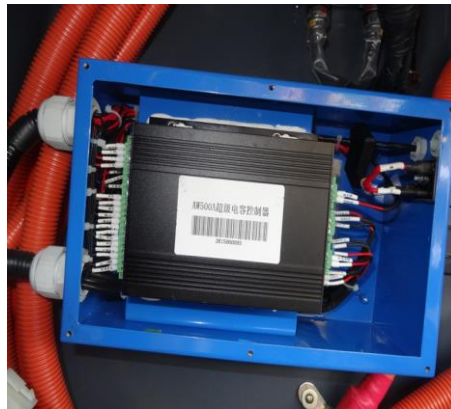
Figure 3 BMS control unit
